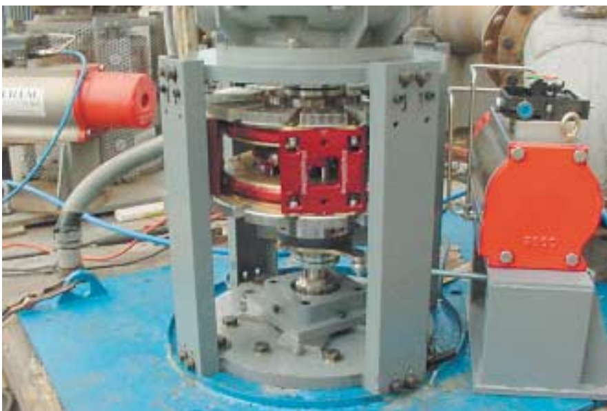
Figure 5: Daishowa America paper mill in Port Angeles, WA, is a typical ASD installation.
