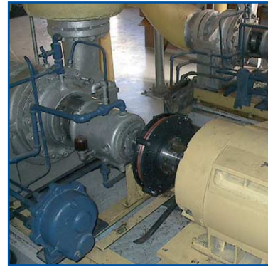
Figure 2. Installation of a PMC between a motor and pump.
